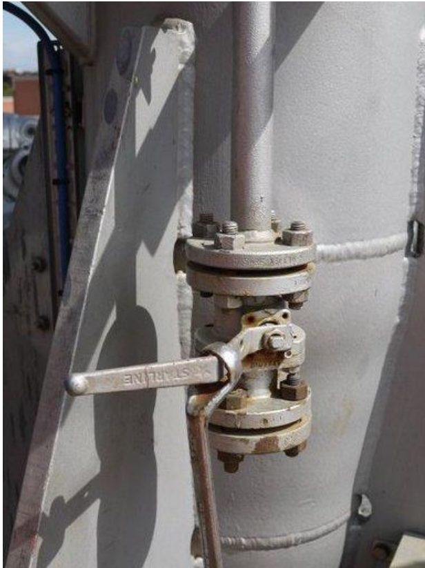
Valve not labelled. Action raised to address
